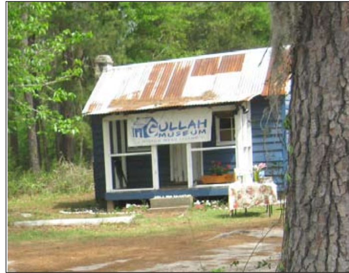
Volunteers worked to preserve the only remaining Gullah home on Hilton Head. They rid the cottage of termites, installed a new roof, replaced rotting beams, and installed a Plexiglas window so visitors could see what a Gullah home of the 1930s looked like inside.
